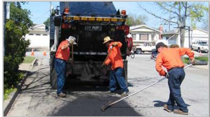
Asphalt patching in residential area
